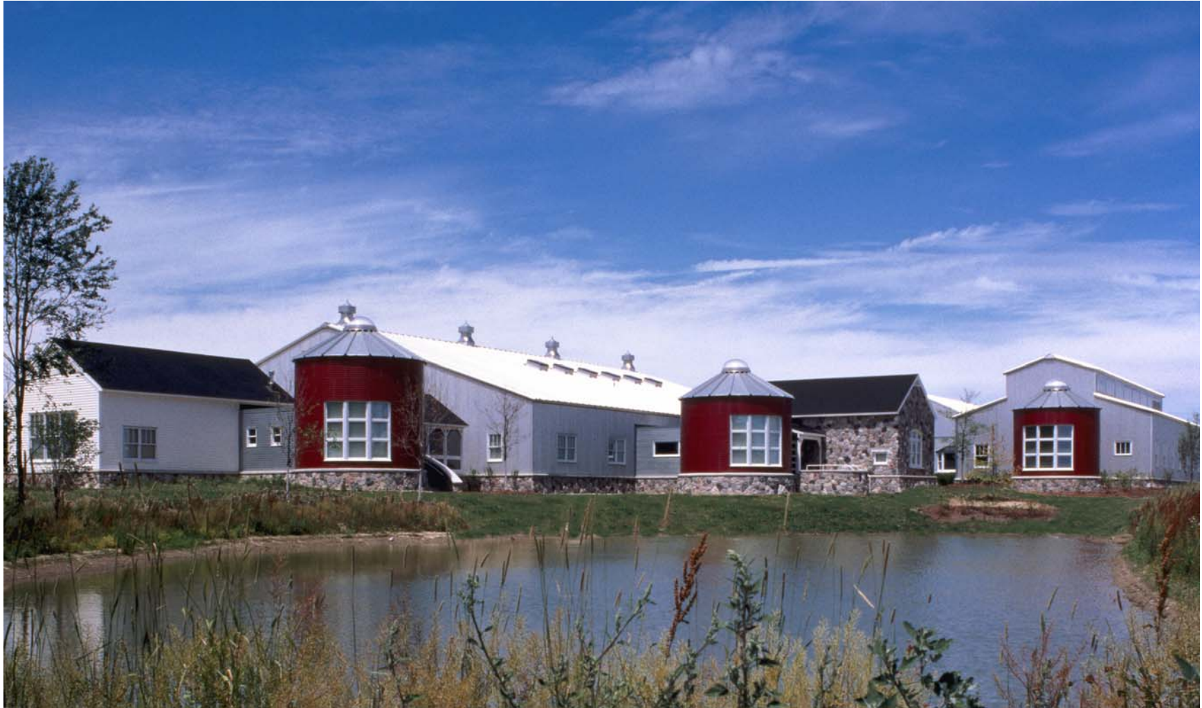
Design Yard facility located in Holland, Michigan.
