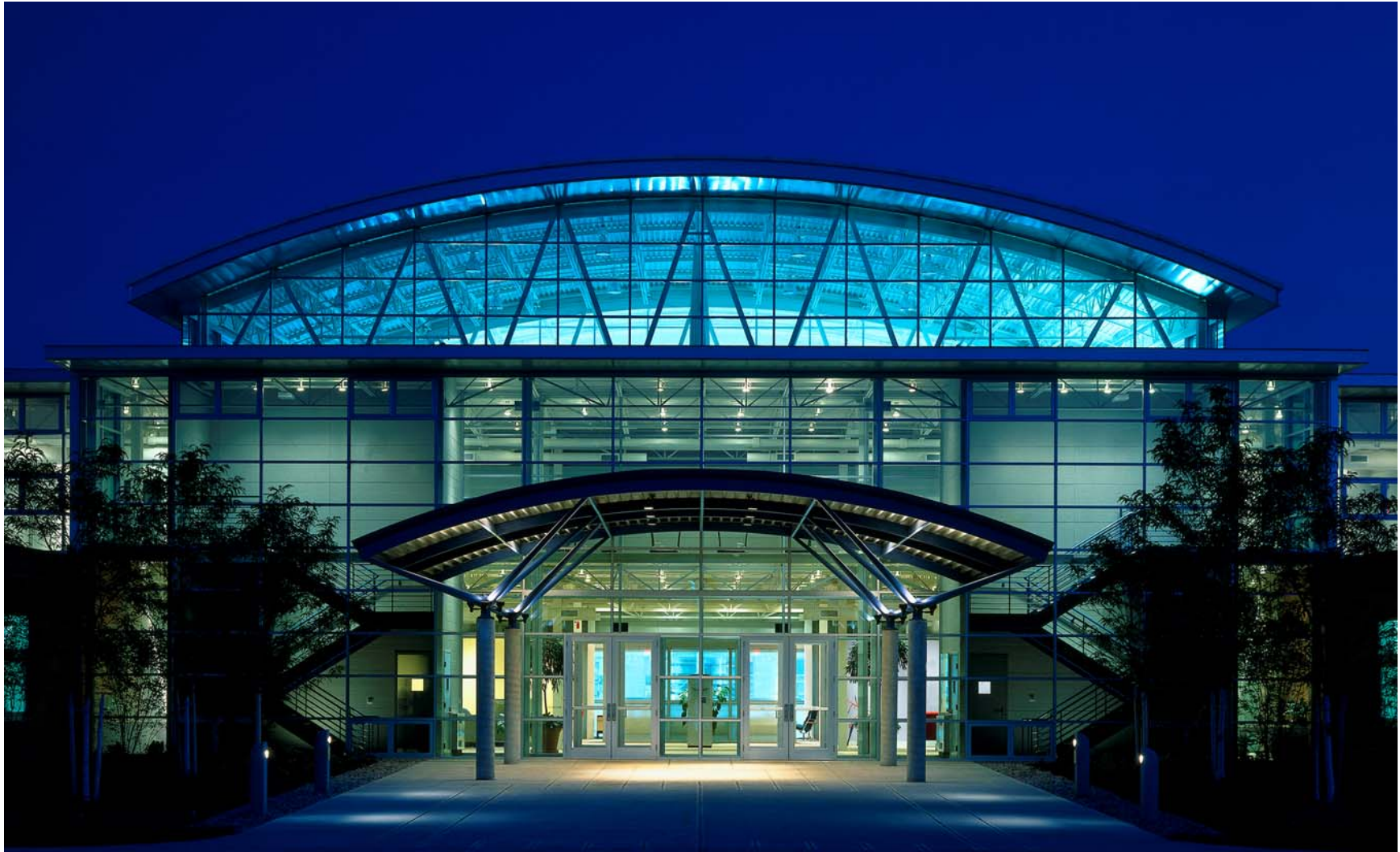
GreenHouse facility located in Holland, Michigan.
