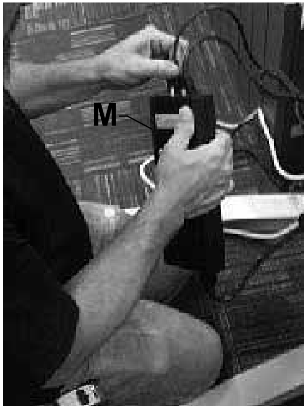
21. Connect lift wiring to Control Box (M).
